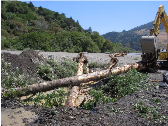
Figure 3 Apex jam under construction
