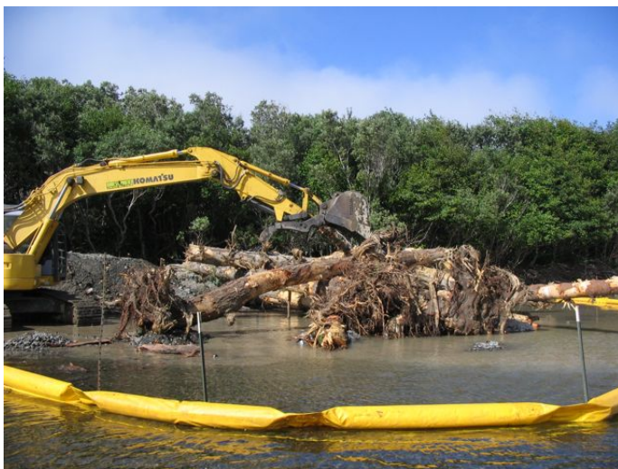
Figure 2 LWD structure #5 under construction
