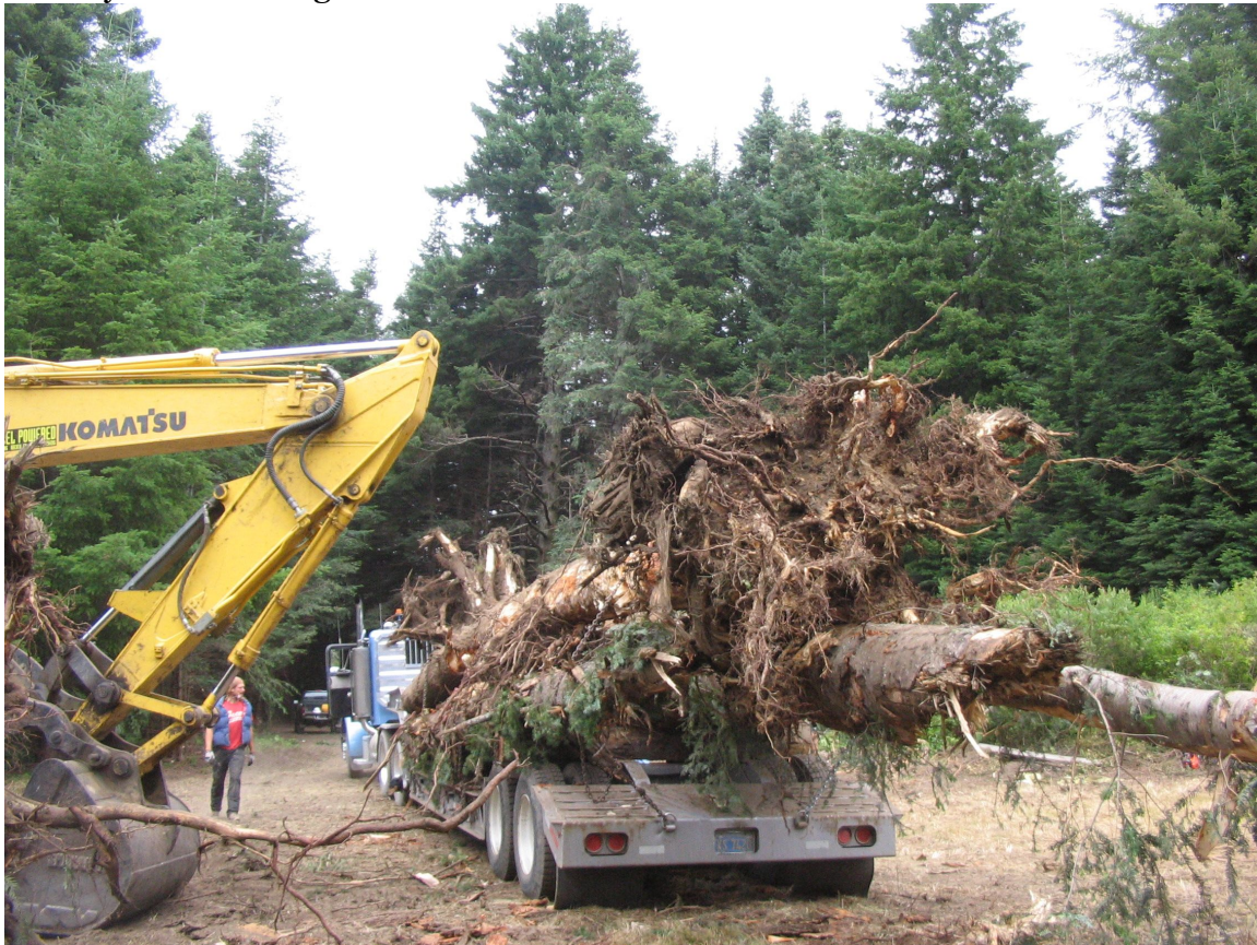
Figure 1, Low-bed ready for haul to Project Deck A
