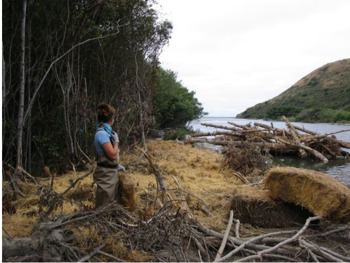
Figure 4 Mulching disturbed sites after construction
