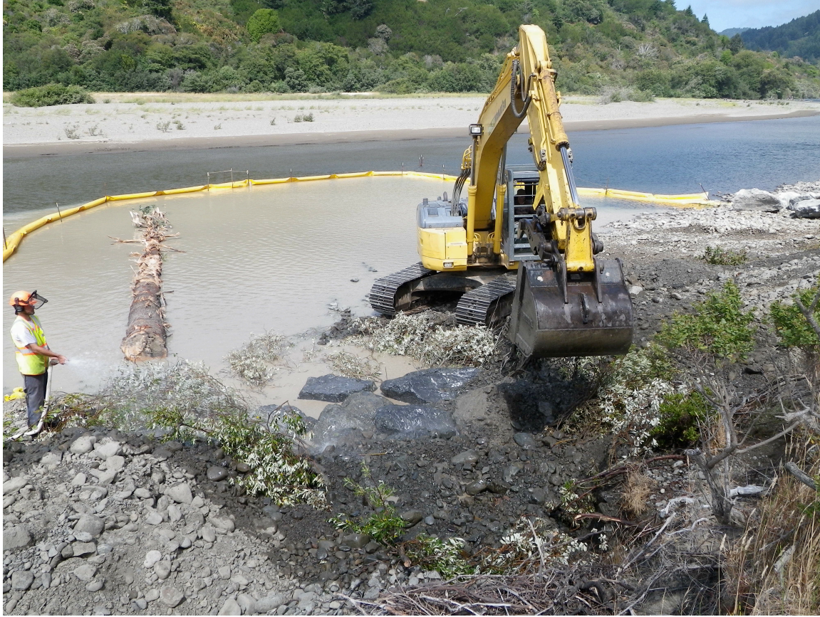
Photo 2. Construction in progress, August 2011
