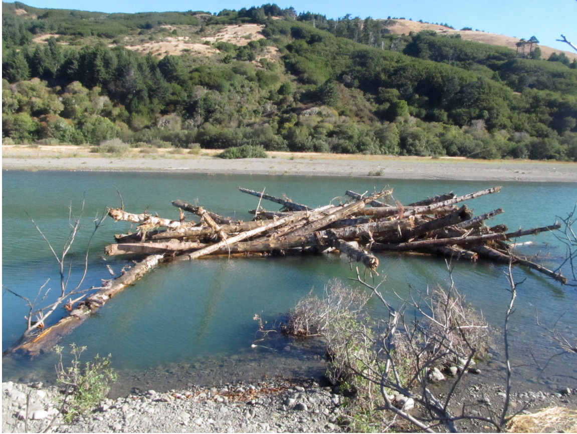
Photo 3. The Completed LWD structure August 2011
