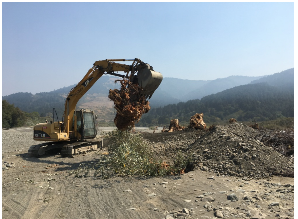
Above: Placing wood in willow trench, 2017. Photograph by Hugh McGee.
