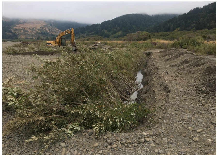
Trenched willow installation, 2017. Photograph by Hugh McGee.
