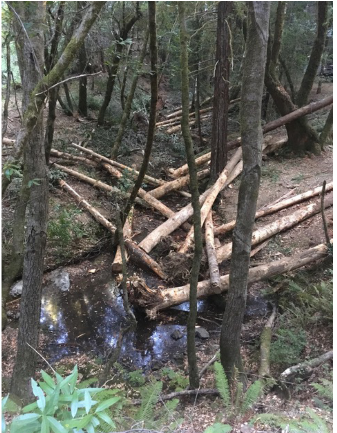
Above: A very complex wood structure located in the mainstem of the Mattole River in Mendocino County. Photograph by Campbell Thompson.
