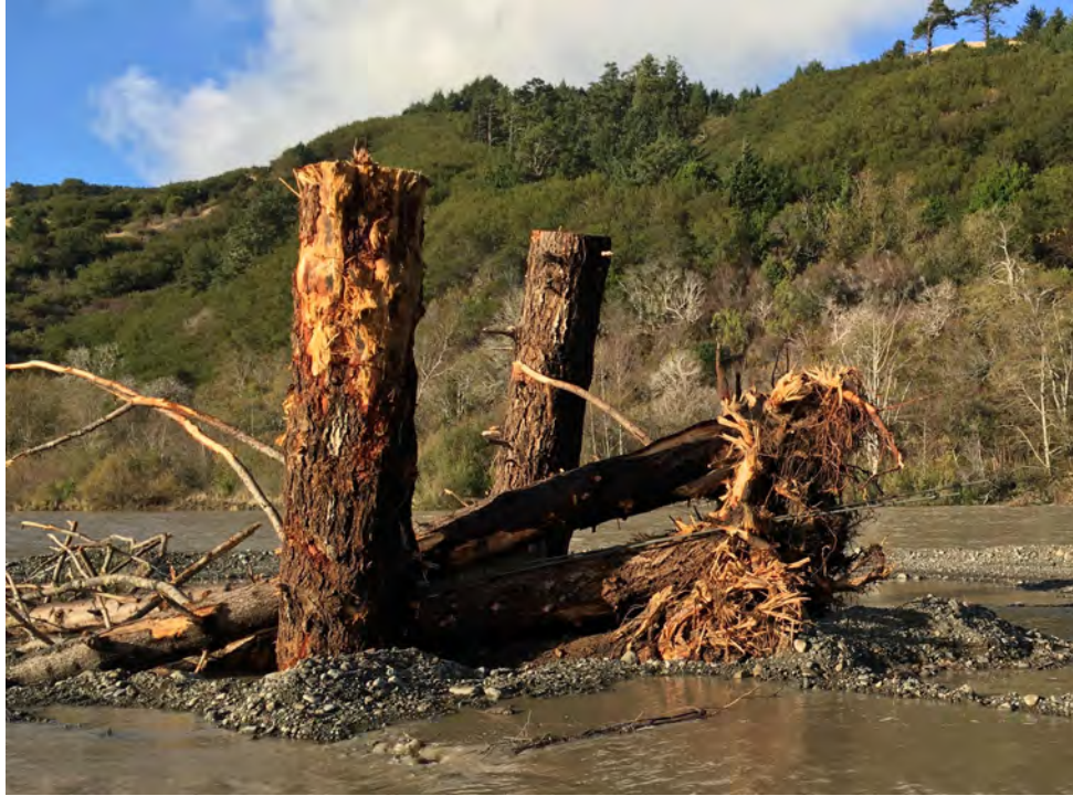
Figure 8. Start of Woodzilla 2 with two 26,000 lb.40 foot long tree boles with root wads
