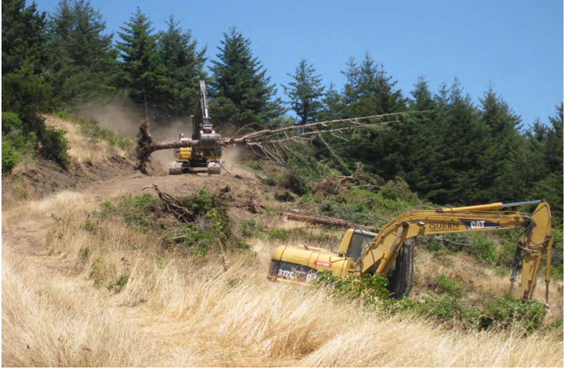
Figure 2. Excavator working deck.
