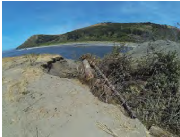
Figure 13. Trenches with willow & wood
