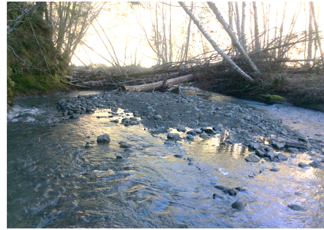
Figure 6. Same view in 2022. This wood structure has captured spawning-size sediment upstream, caused scour of deeper pools along both banks, and will over time continue to add complexity. Photograph courtesy of Mattole Salmon Group
